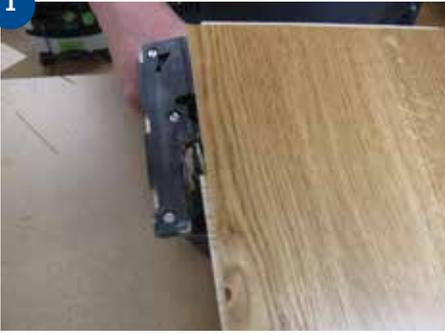
Before installing the first row, the part of the groove profile which sticks out must be cut off.
