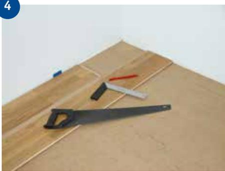
4 Cut the board to the right length with a handsaw (from the top of the board) or a circular saw (from the underside).
