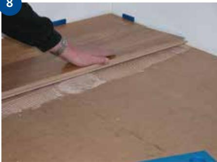
Go back along the row of boards, pressing them down against the subfloor (into the adhesive). Continue as in points 6-8.
