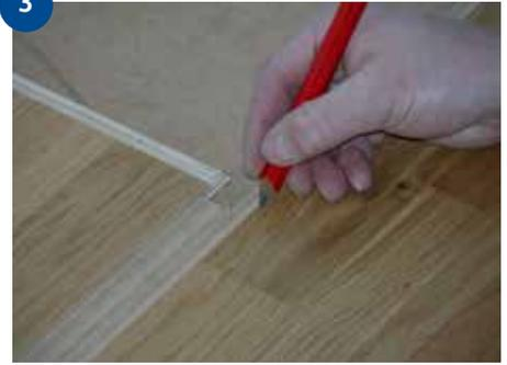
At the end of the row, turn the last board so that it lies tongue to tongue. Push the short end tightly against the wall. With a pen, mark where to cut 8-10 mm from the end of the previous board, to make it easier to get the board into place.
