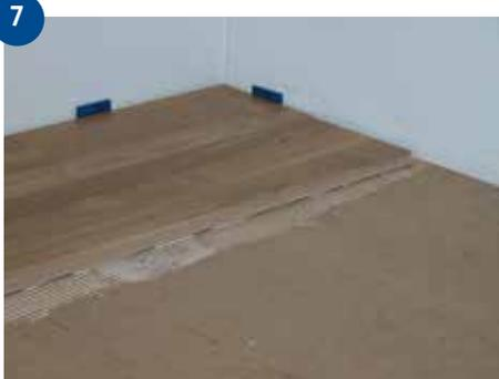
7 Angle the next board into place along the short end. Then push the board until the long side is in place in the groove. Do not press the board down into the adhesive. Continue in the same way with the next board until the whole row is in place.
