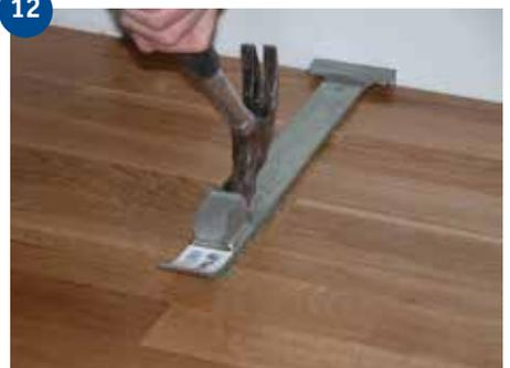
Spread out adhesive, lay the last row of boards and tap them into place using the pull bar.
