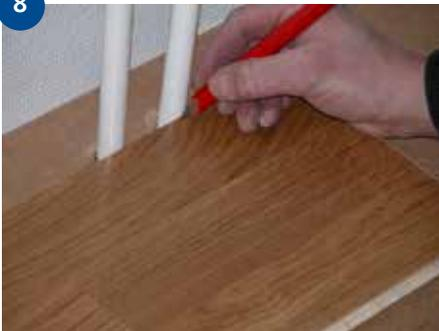
If the long side of the board meets a pipe: Drill a hole with a diameter approx. 10 mm greater than the diameter of the pipe. Measure how far from the end of the board the hole needs to be drilled...
