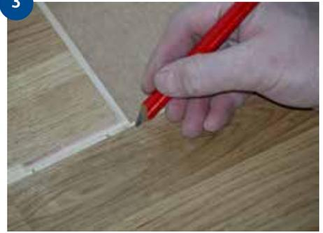
With a pencil, mark where to cut 8-10 mm from the end of the previous board, to make it easier to get the board into place.
