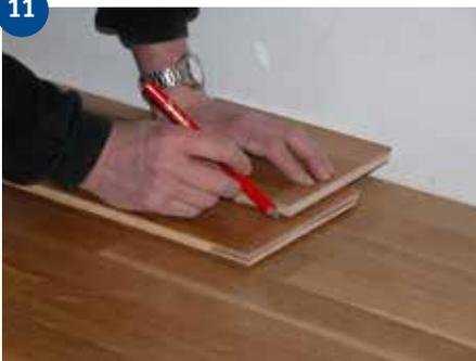
The final row of boards usually needs to be cut along its length. With its tongue against the wall, place the final board exactly on top of the last-but-one board. Place a spare bit of board on top and measure the gap by running the bit of board along the wall and marking with a pencil where to cut the final board.
