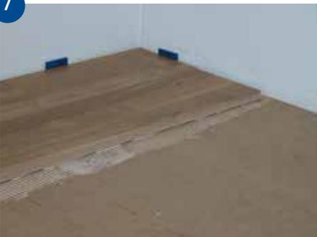
Second plank, second row: Place the panel gently and tight to the short end of the previous panel. Continue in the same way with the next board until the whole row is in place.
