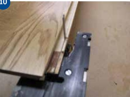
If there is no room to fold down the last board, it can be slid in from the side instead. In order to do this, the tongue of the board in the previous row has to be made level. Use a tool such as a jigsaw or chisel to shave off the part of the tongue which raises like a bump along the top of the outside edge.
