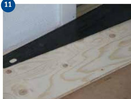
11 Doorframes can be removed and moved up, but it is usually easier to saw them off. Use a loose board as a height template and saw the frame with a fine-toothed saw. Push the floor under the frame. See also point 10.
