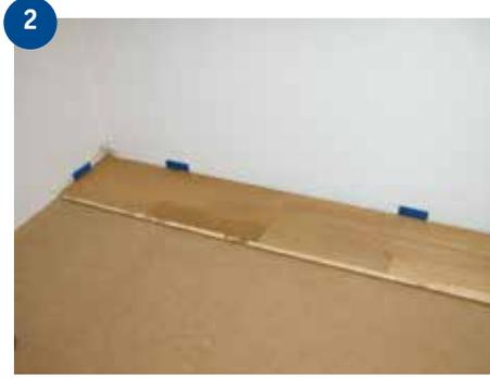
2 Measure out the first row of boards by laying them out without any adhesive.
