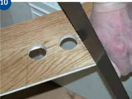
Saw off the bit which will fit behind the pipes, closest to the wall. Cut at an angle as shown in the picture. If the hole is along the short end of the board, cut the board at a 90° angle straight through the hole. Spread out some adhesive and tap the board into place, cover with pipe collars.
