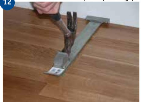
Spread out adhesive, lay the last row of boards and tap them into place using the pull bar and press down.
