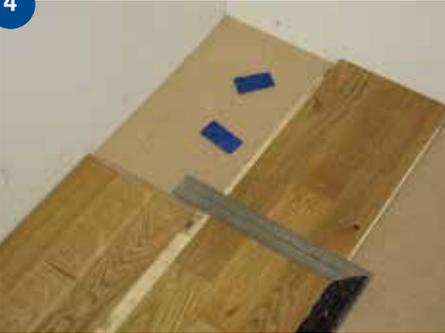
Cut the board to the right length with a handsaw (from the top of the board) or a circular saw (from the underside).
