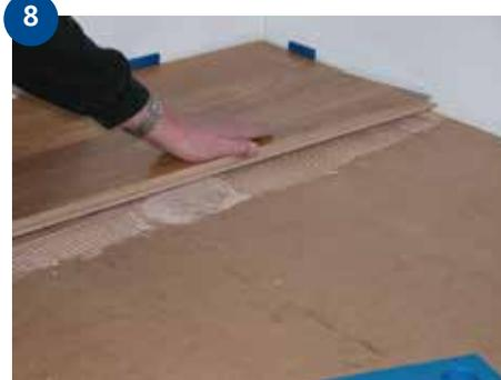
8 Go back along the row of boards, pressing them down against the subfloor (into the adhesive). Continue as in points 6-8.
