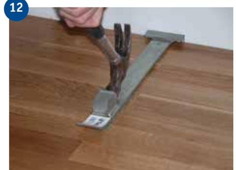
12 Spread out adhesive, lay the last row of boards and tap them into place using the pull bar.
