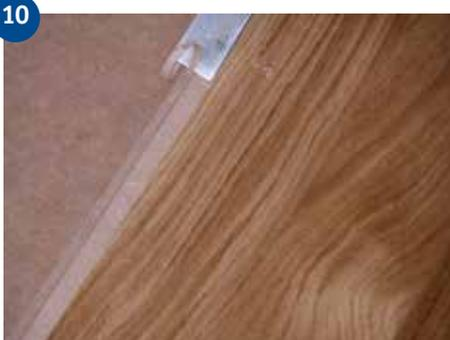
10 If there is no room to fold down the last board, it can be slid in from the side instead. In order to do this, the tongue of the board in the previous row has to be made level. Use a tool such as a chisel to shave off the part of the tongue which raises like a bump along the top of the outside edge.
