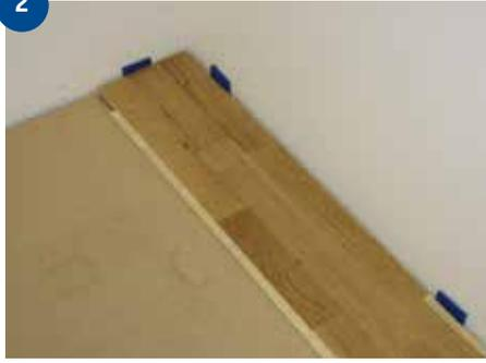
Measure out the first row of boards by laying them out without any adhesive.
