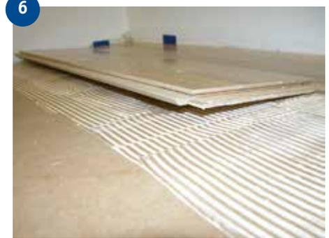
6 Repeat points 2-4, take up and spread adhesive. Start the second row with the rest of the board cut from the first row. Lay the board in place in the groove without pressing it down.
