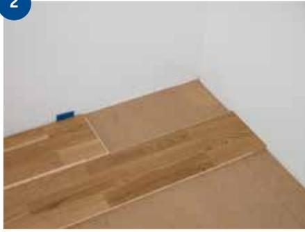
At the end of the row, turn the last board so that it lies tongue to tongue. Push the short end tightly against the wall.
