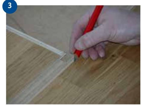
3 At the end of the row, turn the last board so that it lies tongue to tongue. Push the short end tightly against the wall. With a pen, mark where to cut 8-10 mm from the end of the previous board, to make it easier to get the board into place.
