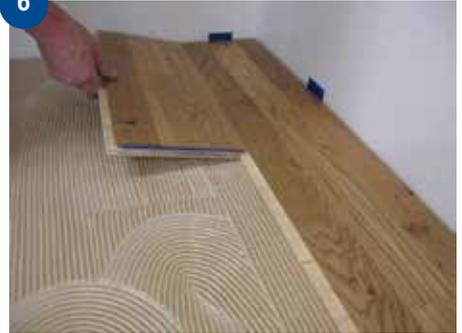
Repeat points 2-4, take up and spread adhesive. Start the second row with the rest of the board cut from the first row. Lay the board in place in the groove and press down.
