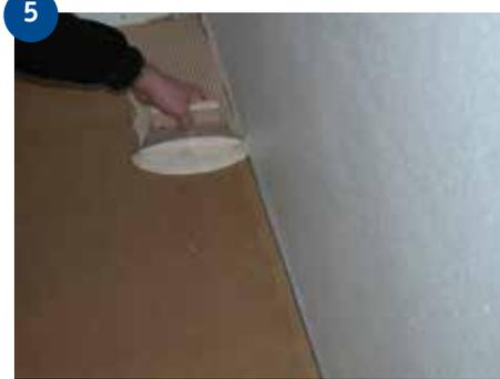
5 Take up the row of boards you laid out. Spread adhesive over the subfloor where the whole row of boards will lie. Lay the boards down one by one and wedge them against the wall.
