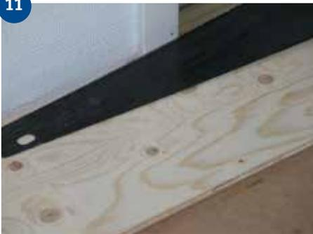
Doorframes can be removed and moved up, but it is usually easier to saw them off. Use a loose board as a height template and saw the frame with a fine-toothed saw. Push the floor under the frame. See also point 10.
