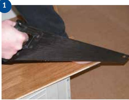
1 Before installing the first row, the part of the groove profile which sticks out must be cut off.
