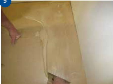
Take up the row of boards you laid out. Spread adhesive over the subfloor where the whole row of boards will lie. Lay the boards down one by one and wedge them against the wall.
